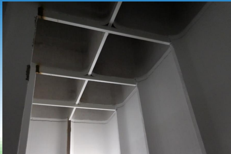
Flour storage bins have rounded corners.
