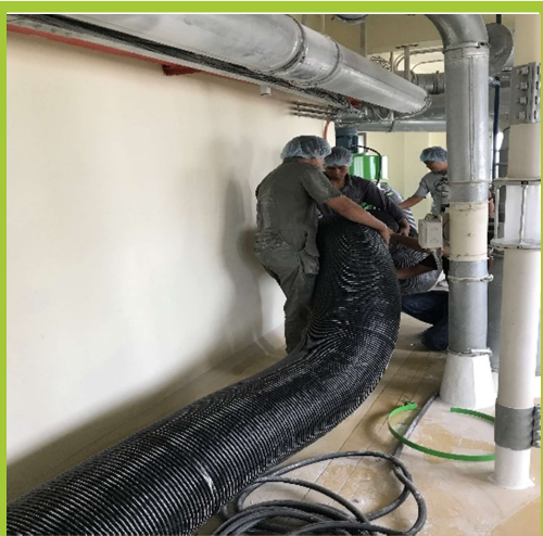
Connection of flexible duct
