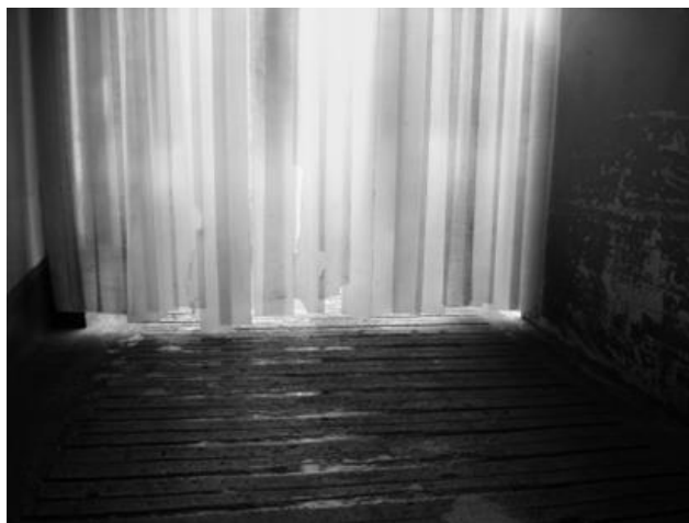
Fig. 2. Damaged bottom of plastic strip doors allows pest entry
